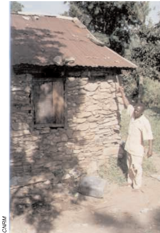
Mzee Lukuyu pointing at the damaged roof from contaminated rain next to Webuye paper factory.
